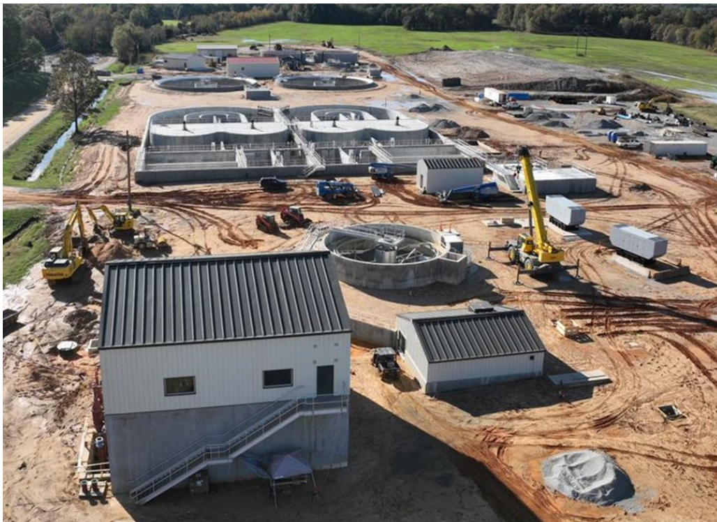
Figure 4-1: Construction of Westside WWTP Structures (October 2023)
